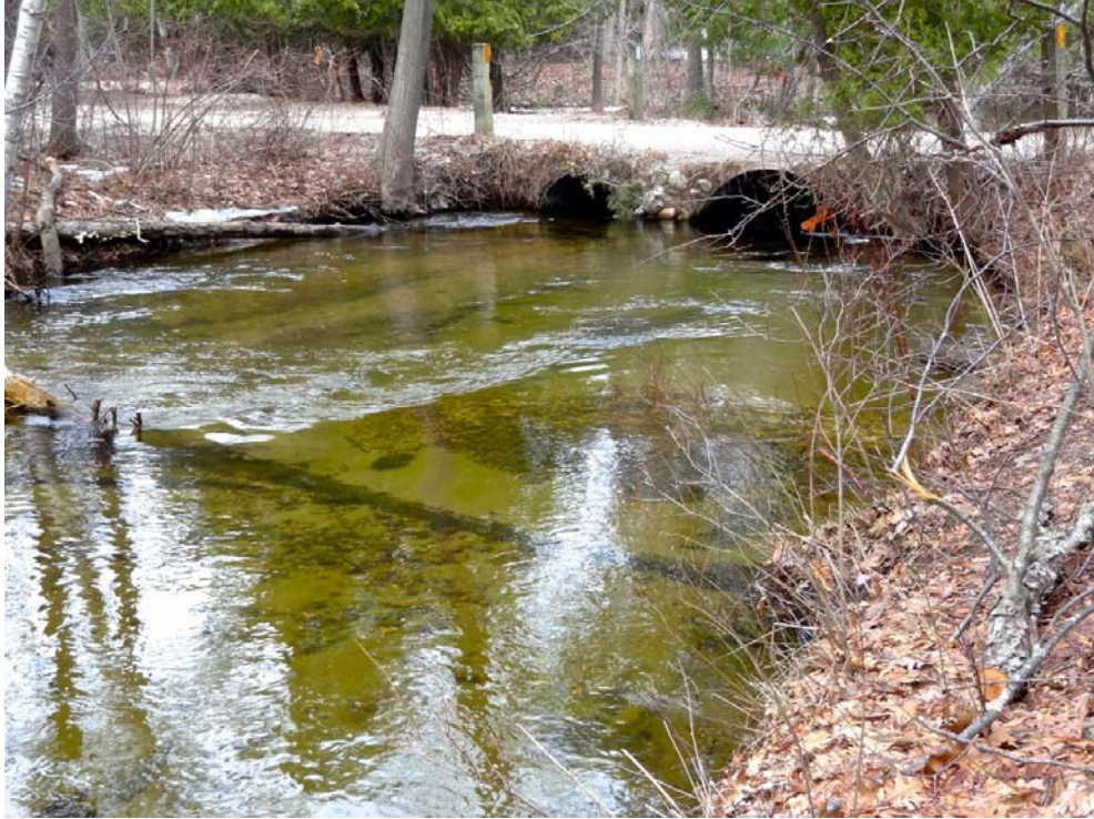
Figure 10: 2014 photo of Culvert -County Road 669 (Shalda Creek Crossing), looking upstream
